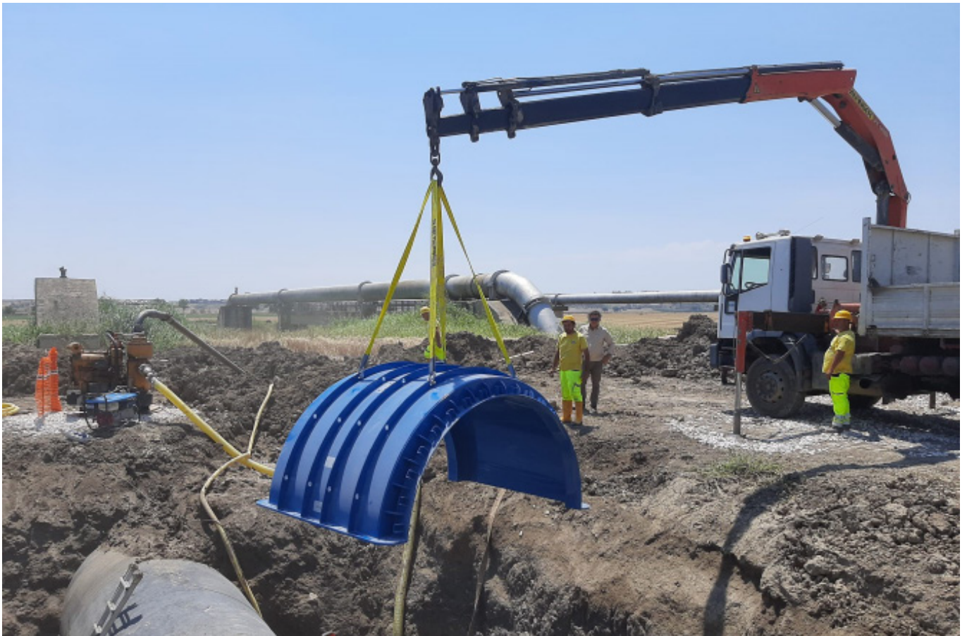
The DN2000 collar being installed
