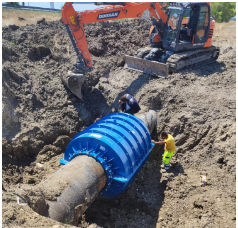
The DN1000 collar being installed
